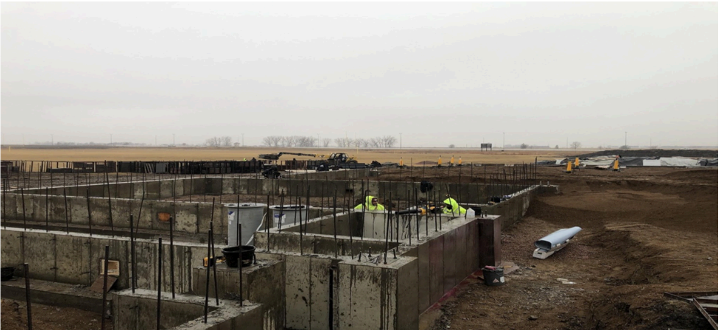
December 30, 2024: foundation walls poured, including the elevator shaft (in front of the workers).
